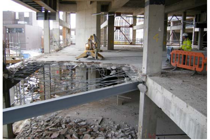
Swathe cutting works on the double height mall
