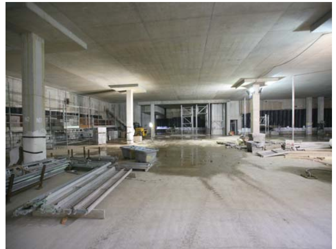
Debenhams basement area
