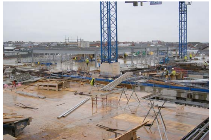
Erection of roof steel on the plant deck
